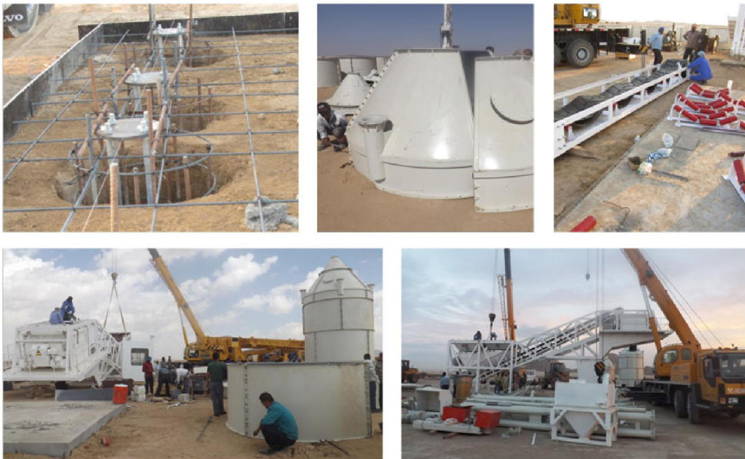
Installation of YHZ60 mobile concrete mixing plant
